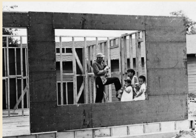
Flanner House self-help housing construction, early 1950s
